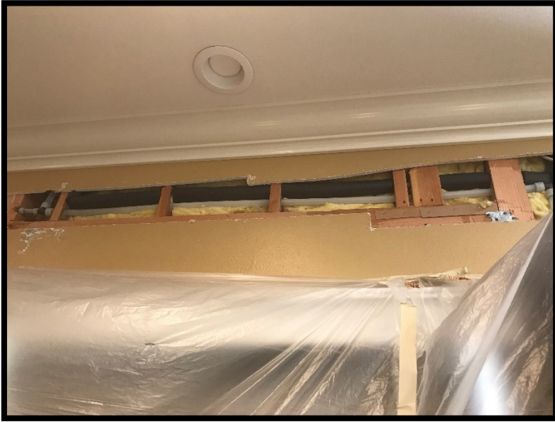
Remove Drywall and install Pex Pipe
