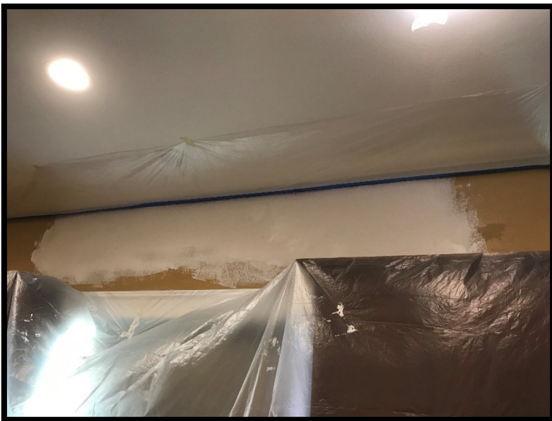
Texture drywall, prepare for paint
