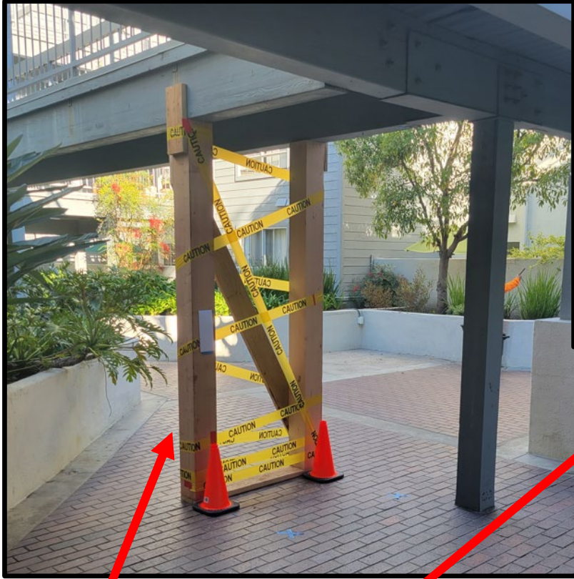
Emergency shoring to prevent collapse
